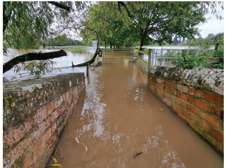
Flooding at the old bridge
